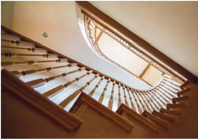
A focal point of the entry, the hand-crafted, cherry stairway, made at Dietz Designer Cabinetry and assembled onsite, required precise measurements and attention to detail.
